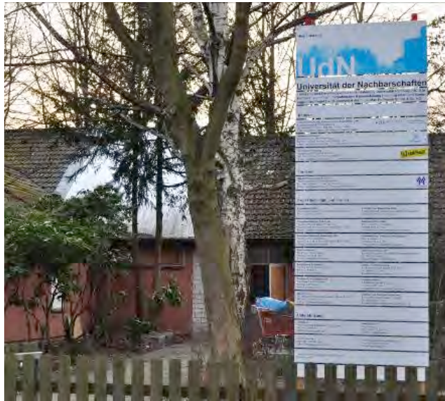
Figure 4 | Construction site panel of the UdN building inside the island of Wilhelmsburg
