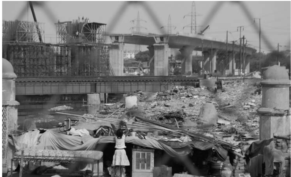
Picture 8. Pre-Commonwealth Games works in progress
