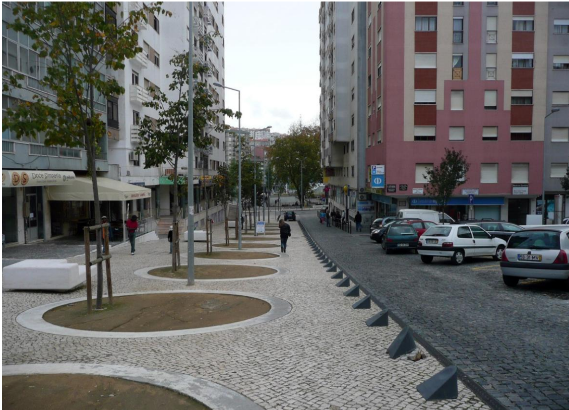
Figure 4. Cacém Polis Public Space .D. Maria II Street after the intervention (photography by the author).
